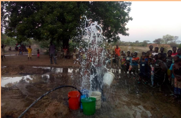
They hit water at 45' and it is giving 9,000 liters per hour.
