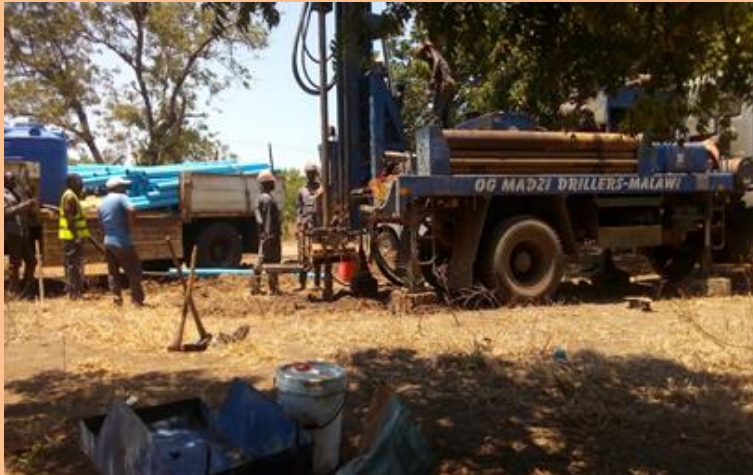
Well drillers arriving at Tengani
